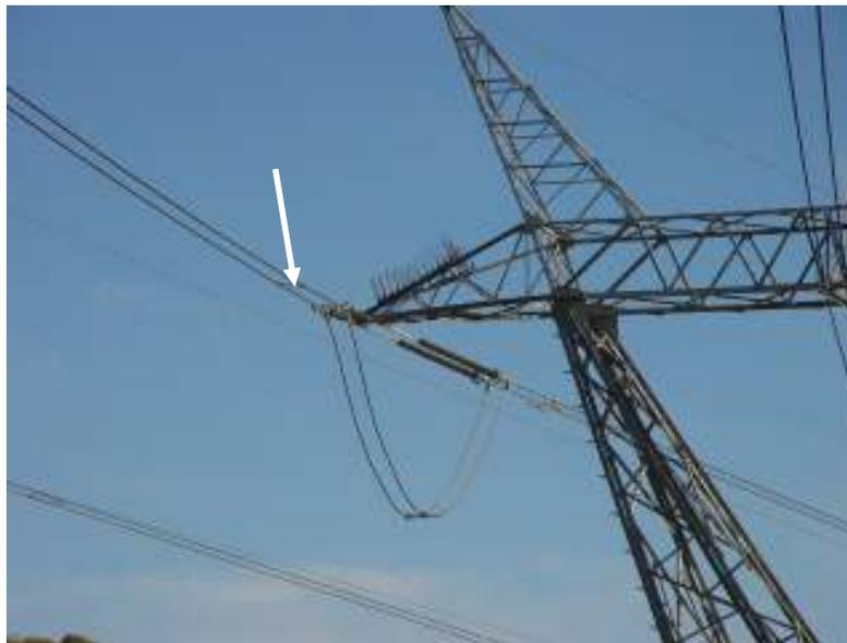
Picture of incorrect fitting leaving the landing plates exposed
