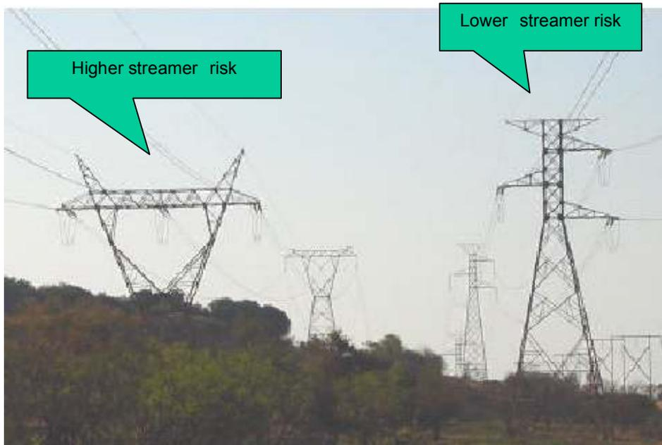
Horizontal strain towers are the most vulnerable to streamer faults, followed by horizontal suspension towers. Delta towers are generally much less vulnerable with suspension towers being the least vulnerable.
